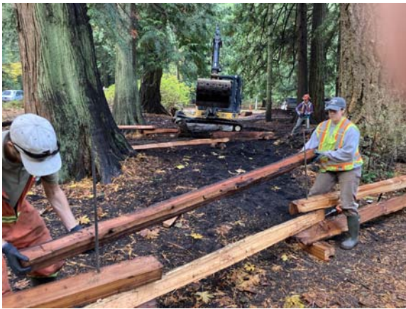
A new split rail fence for the planted area
