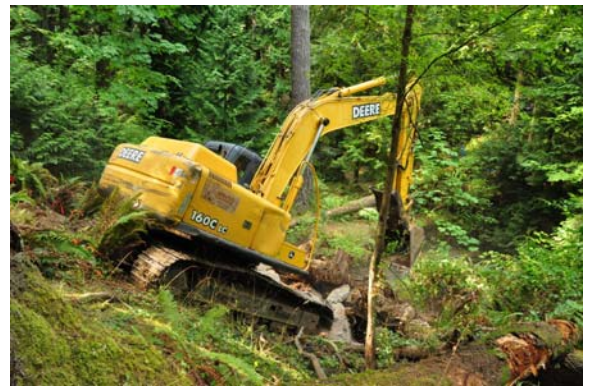
Placing root balls & logs on the creek bank
