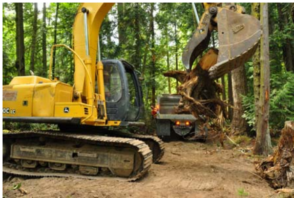
Root balls are transferred to creek.
