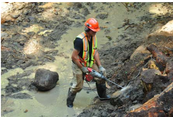
Drilling for anchor cables
