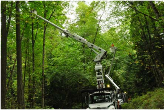
Two boom trucks used to access dead, overhanging branches.
