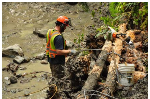
Cables around logs to protect creek banks.
