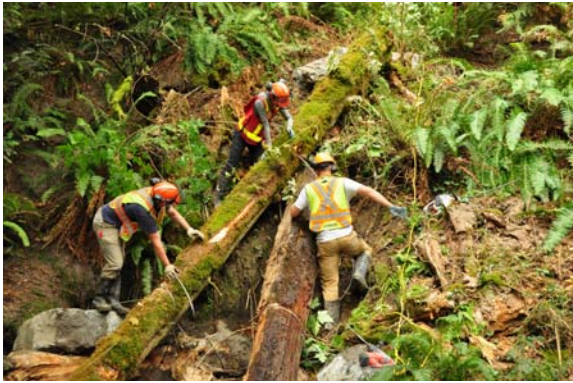
Logs and tree root balls must each be cabled in place to prevent washout from storm surges.
