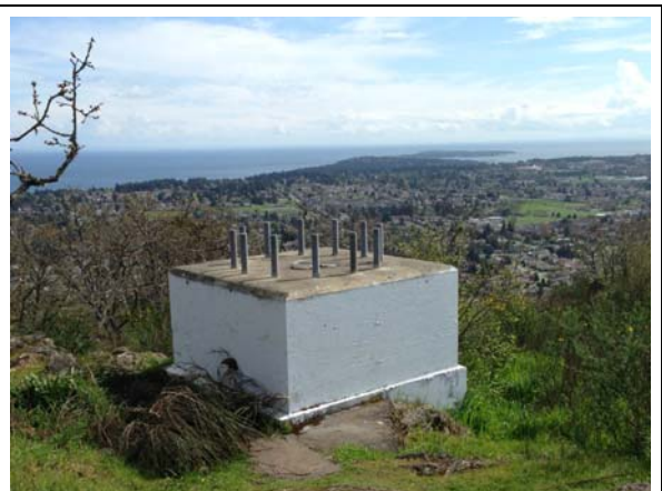
Old unused tower base has to go!
