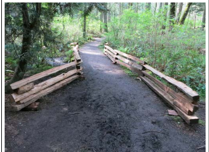
New split cedar fence protects stream crossing
