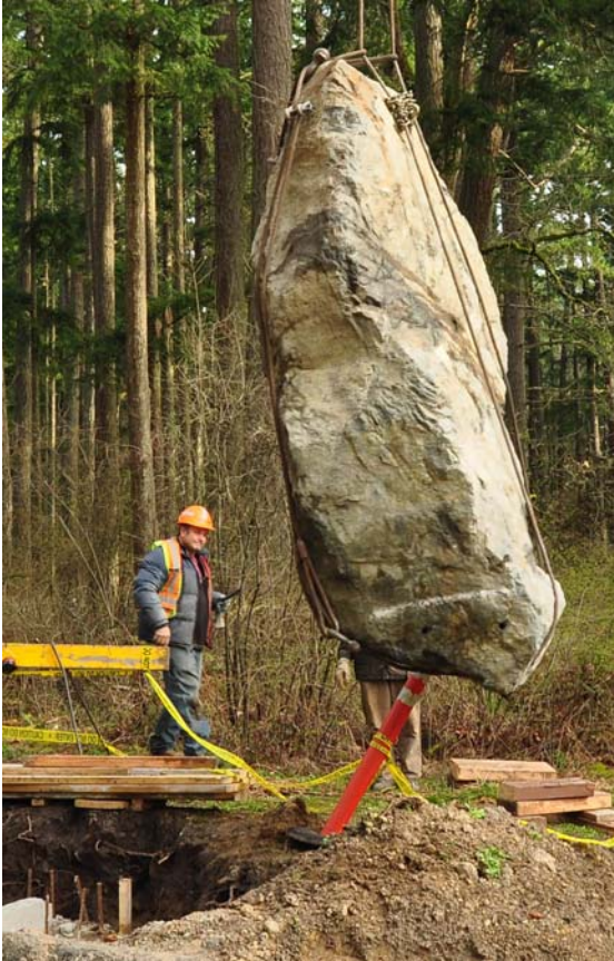
Installation of Entrance Rock
