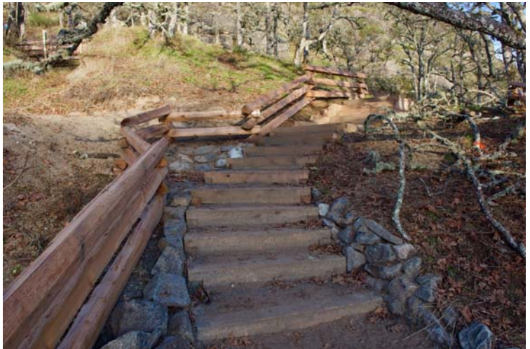
Steps constructed over steep loose sand section. Split rail fence keeps walkers on trail and protects adjacent sand allowing for recovery.
