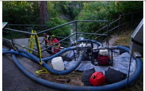
All creek water must be pumped around restoration area during work.
