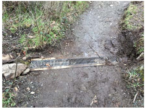
Water bar recently installed on Glendenning Trail near summit.
