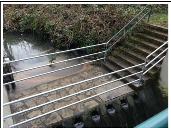
New safety railings at the weir
