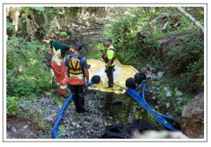
Saanich staff set up a baffle to protect the stream bed from the flow from pumps draining the weir pond.
