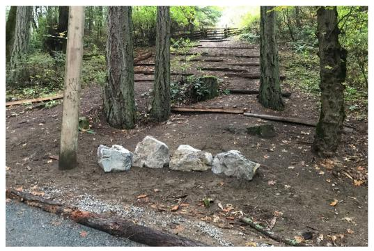
To help reduce the effects of erosion, Whittaker trail, a particularly steep and busy trail in the park, has been partly resurfaced with gravel and water diverters (humps) have been built. A steep slope on the north side of Whittaker, badly eroded by people, has also been reinforced and will be replanted this winter.
