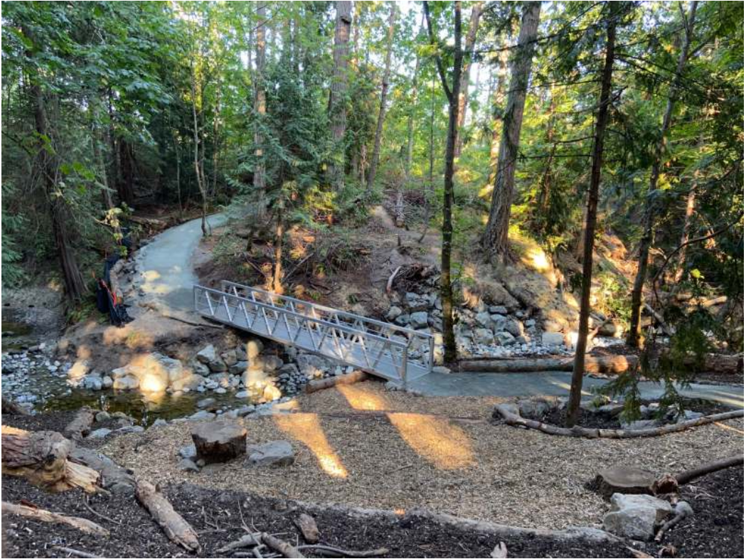
The new bridge over the creek in Mount Douglas Park is ready for foot traffic.
