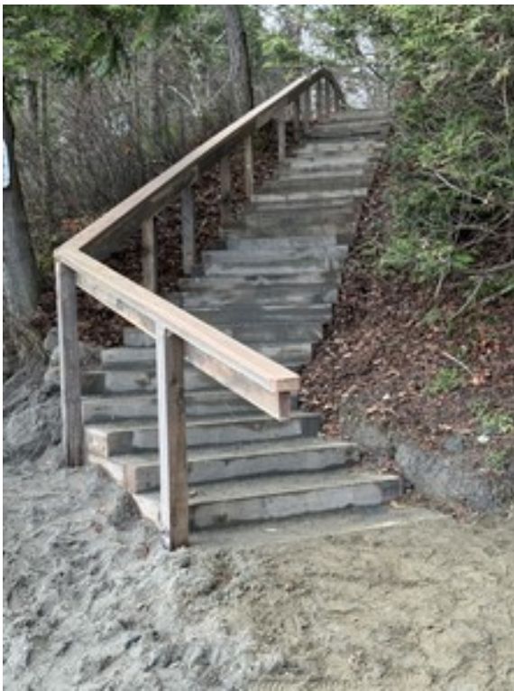
Completed new stairs to the beach
