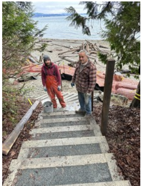
Carpenter Joshua and Bear installing railing for completed stairs
