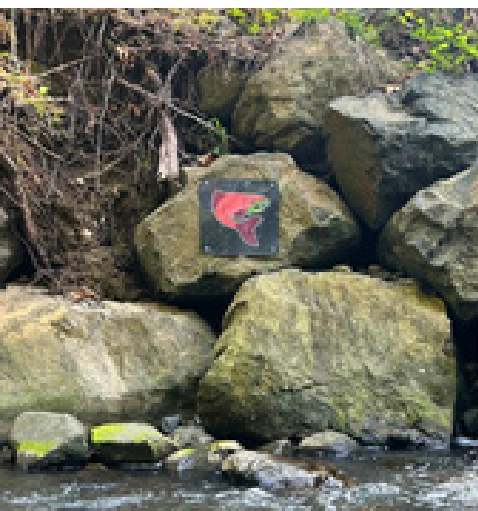
The high-water marker beneath the Douglas Creek Bridge may need to be raised!
